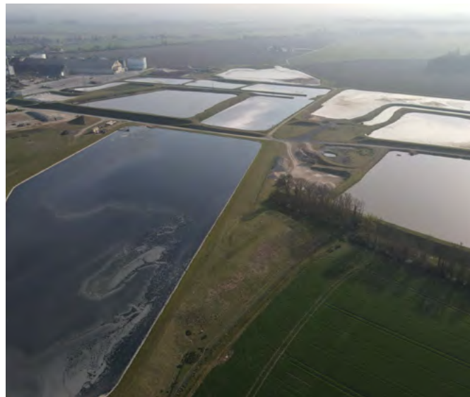
Bassins eau Corbeil © Cristal Union
